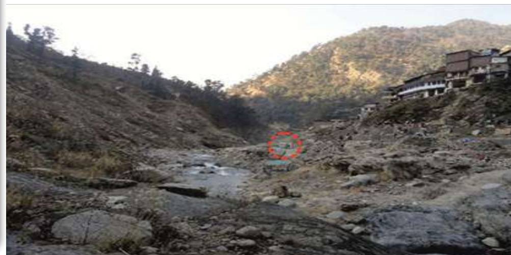
Fig. 1. (a) Gaurikund pre disaster view (b) Gaurikund post disaster view
