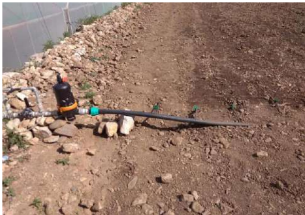
This photograph shows the installation of main line of subsurface drip irrigation with water filter, venturi injector and control valve
