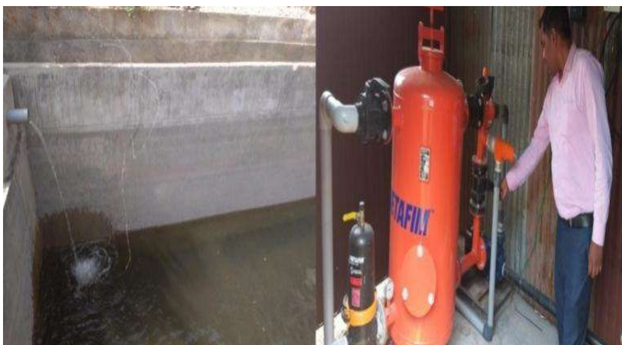
This photograph shows a water tank that is constructed and linked to an electric pump with pre-filter
