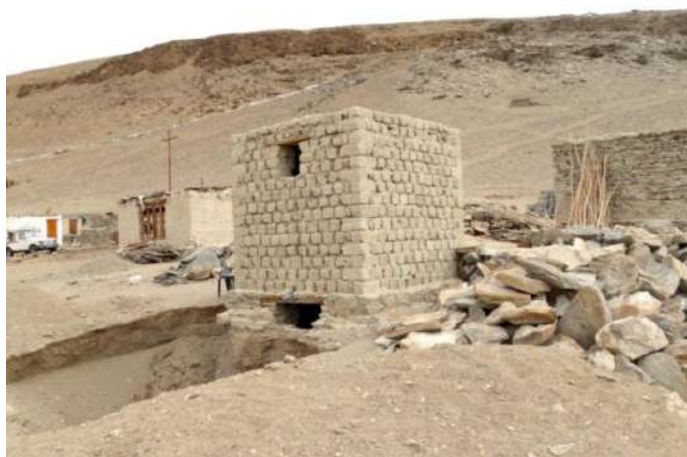
Fig.2: An ongoing construction of a dry toilet ( Source: https://roundglasssustain.com )
