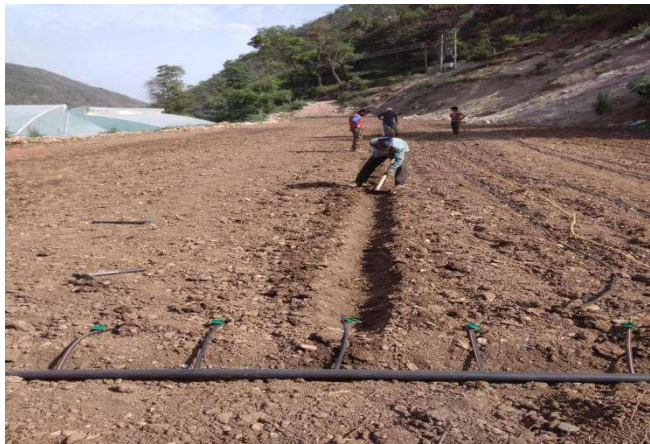
This photograph depicts the labours are making optimum depth (15 cm) for installation of dripnet PC (lateral pipes)
